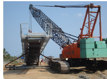
Figure 15: Rock Loading Jetty: Rock transport and large crane
