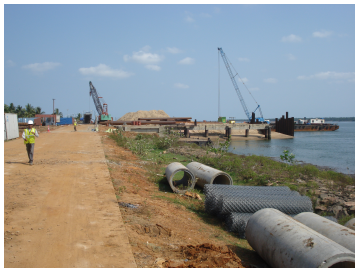
Figure 13: Rock Loading Jetty: road to Jetty
