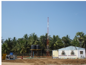
Figure 14: Rock Loading Jetty: Office
