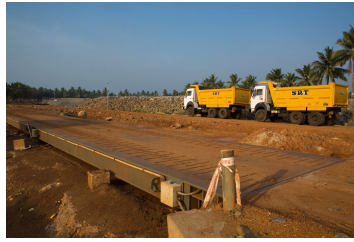
Figure 17: Rock Stockpile: Weigh bridge for the stone trucks
