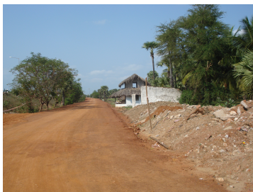
Figure 19: Formation of temporary access road
