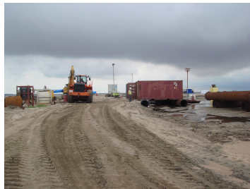
Figure 26: Dry Dump: Equipment on the island
